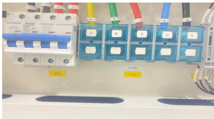
External interface TP 4-PV access, QF 9 battery output switch:
