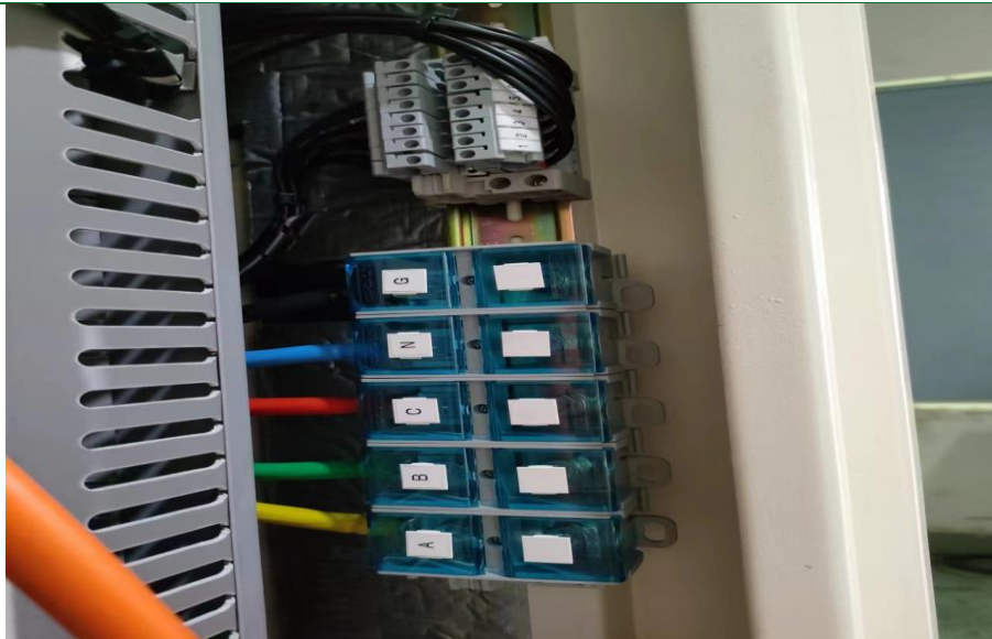
External interface TP 3-load access, TP 5 battery output:
